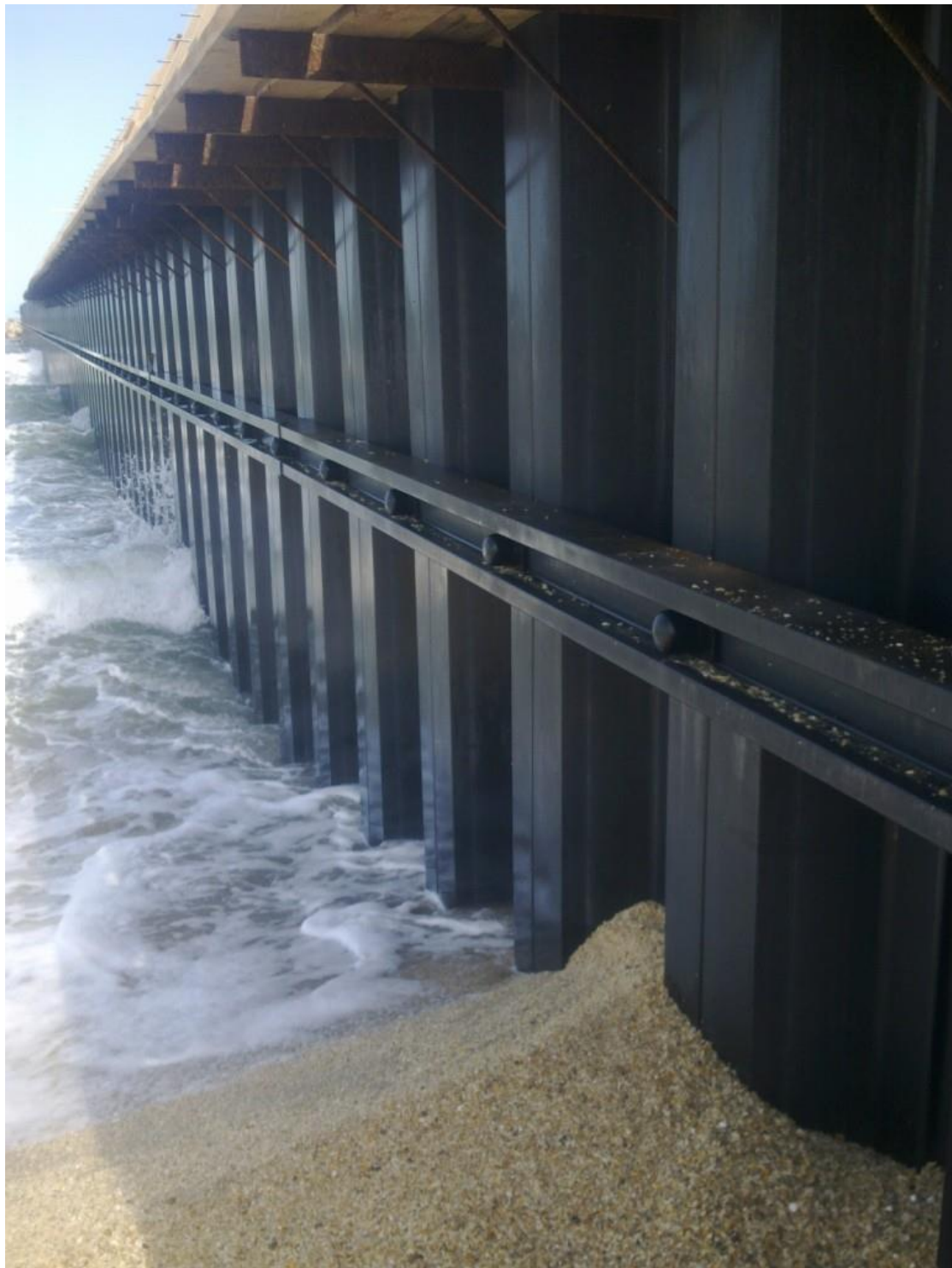
板樁護岸 (steel-pile seawall)
